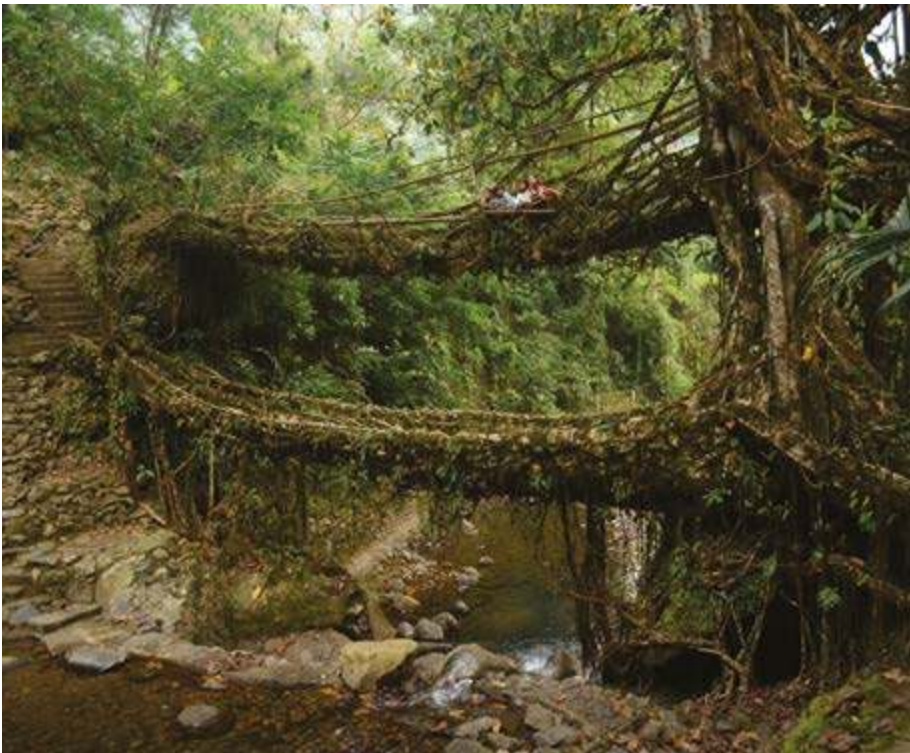
Living root bridges of Nongriat village in East Khasi Hills district (2014). Photo by Pjeganathan, CC BY-SA 4.0, https://commons.wikimedia.org/wiki/File:Living_root_bridges_of_Nongriat_village_in_East_Khasi_Hills_district,_Meghalaya_JEG7363.jpg
