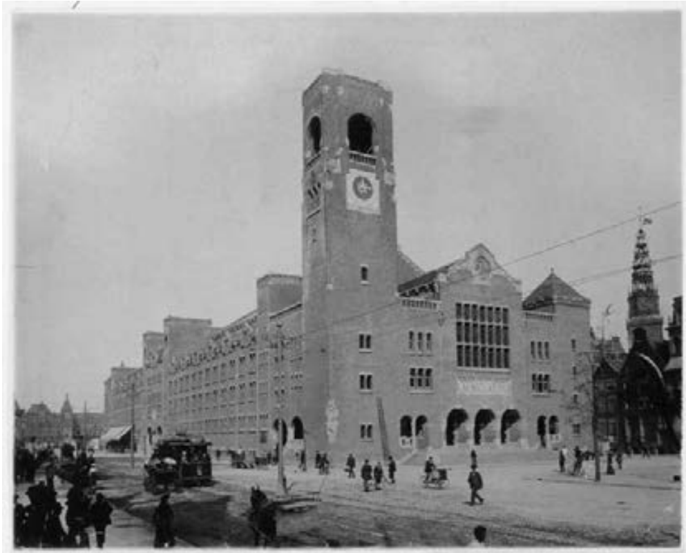
Figure 2.3. The modern world of commerce and technology was steeped in a Renaissance aesthetic. Berlage had been commissioned to build a new stock exchange in the 1885. The construction work started in 1898, and the building was revealed to the public in 1903.
