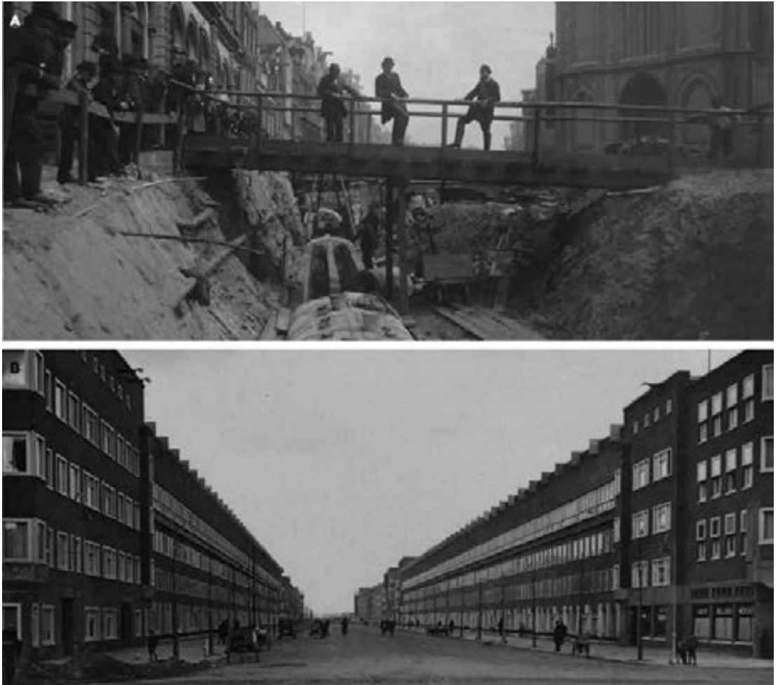
Figure 2.2. (A) The draining of canals opened up the possibility of implementing new technologies underneath the city's skin. Here a sewage system was installed on the Nieuwezijds Voorburgwal in 1884. (B) Berlage and his peers introduced modern, straight streets to Amsterdam. This image shows the Hoofdweg in 1920.
