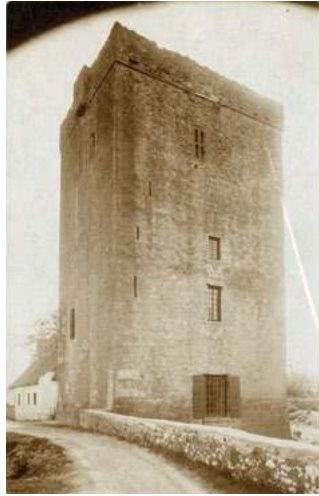
Plate 23b. Photograph sent by Yeats to Sturge Moore of Thoor Ballylee, to be used as the basis for the design in Plate 23a. The back is inscribed 'The cottage at back is my kitchen. The front you will see is over parapet of the old bridge. The other [parapet] was blown up during our civil war. WBY'. © Senate House Library, London. All rights reserved.
