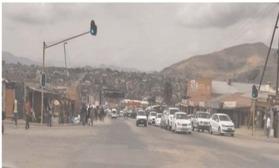
Figure 2. Unmarked intersecting roads.
