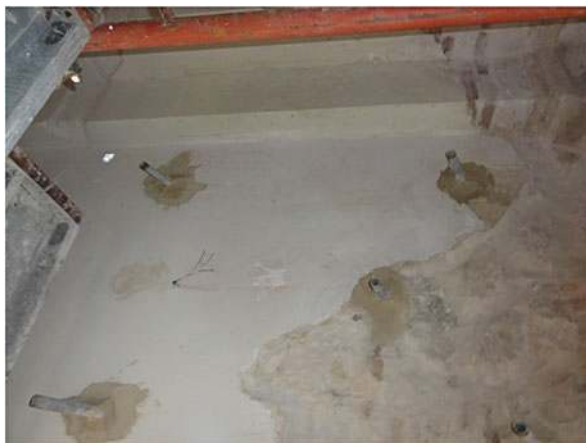
Fig. 15.6 Wall prepared for grout injection
