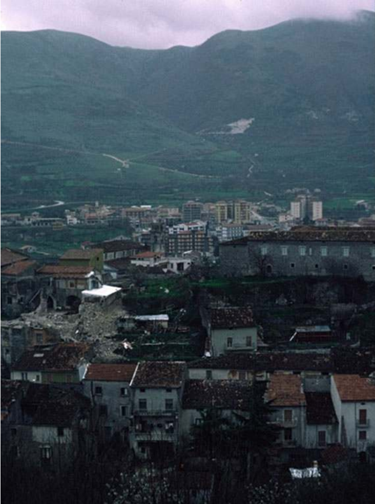
Fig. 1.6 Polla from the same location as Fig. 1.6 in 1981 after the Irpinia earthquake. Note similarity of building form and construction (Photo by author)
