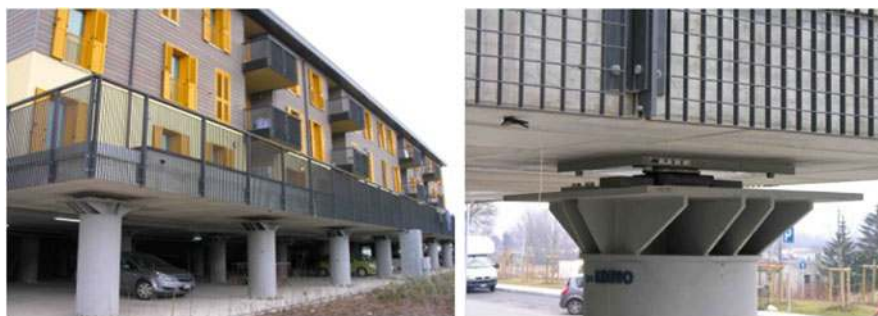
Fig. 14.20 Left : one of the 184 pre-fabricated houses (wood, or r.c., or steel structures) erected in L'Aquila to host up to 17,000 residents who remained homeless after the 2009 Abruzzo earthquake. Right : detail of one of the 40 CSS devices, manufactured in Italy, which have been installed at the top of columns (made of steel or r.c.) to isolate the supporting slabs of such houses
