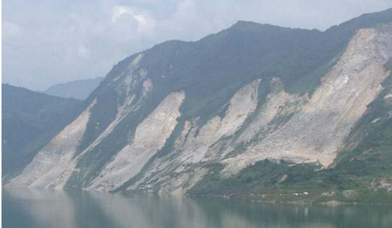
Fig. 20.3 Rockfalls in the Zipingpu reservoir area caused by the 2008 Wenchuan earthquake in China
