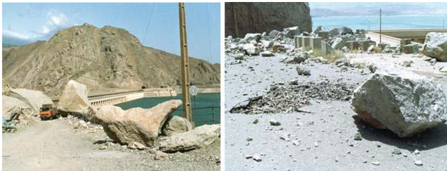
Fig. 20.6 Access roads to Sefid Rud dam site blocked by numerous rockfalls caused by the 1990 Manjil earthquake in Iran
