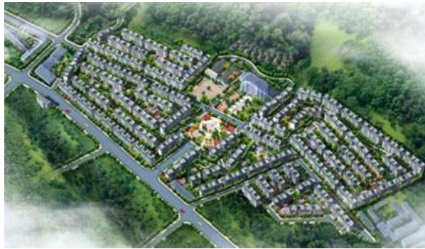
Fig. 14.8 Complex of dwelling buildings in South-Western P.R. China, formed by 94 4- to 6-storey seismically isolated buildings (overall floor area = 280,000 m 2 ) (Eisenberg et al. 2011)
