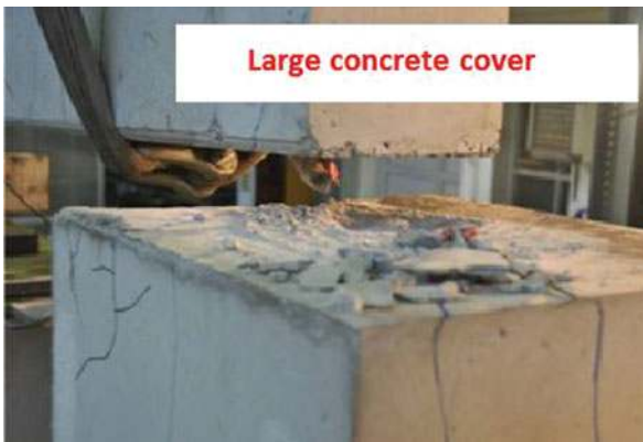
Fig. 4.33 Rupture of the dowel in the case of large concrete cover
