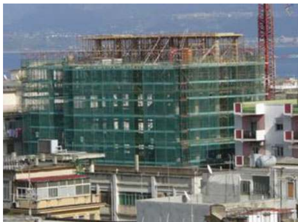
Fig. 14.19 Eight-storey isolated building which is nearing completion in Messina on 22 LDRs and 2 SDs. Its structural safety will be certified by A. Martelli in 2014
