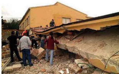
Fig. 14.14 Francesco Jovine school of San Giuliano di Puglia, after its collapse during the 2002 Molise & Puglia earthquake ( M = 5.9 )
