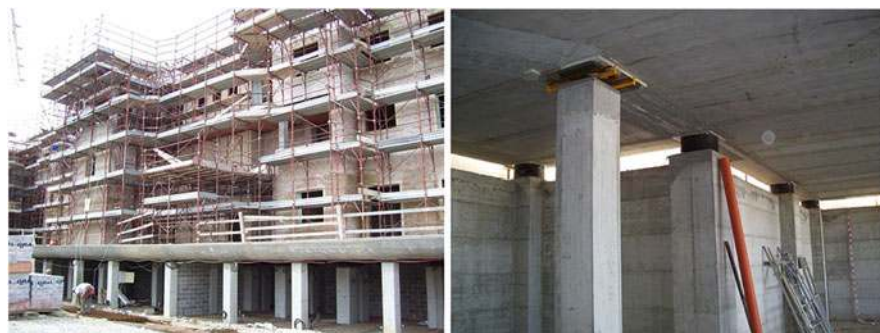
Fig. 14.24 Left : seismically isolated dwelling building complex under construction in Ozzano Emilia (Bologna), irregular in shape (61 m \times 28 m; 2 buildings with 2 staircases, connected to the second floor; 4 isolated above ground isolated floors, with the isolators installed in the non-isolated basement). Right : some of the isolators of the building (61 HDRBs and 56 SDs)
