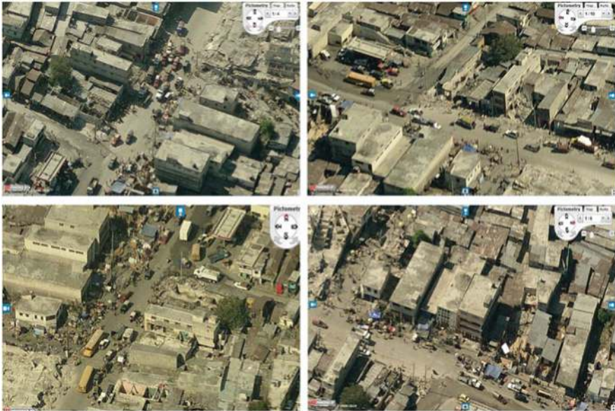
Fig. 1.19 Pictometry images of damage in the 2010 Haiti earthquake (Booth et al. 2011a)
