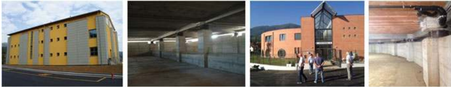
Fig. 14.30 Left : one of the 2 isolated blocks of the new primary and secondary school of Galliciano (Lucca, Italy), former seismic zone 2, which was erected with the collaboration of GLIS and was opened to activity in September 2009. Centre-left : some of the 46 HDRBs installed in their underground floors. Centre-right : the new isolated kindergarten and primary school of Mulazzo (Massa Carrara, Italy), former seismic zone 2, certified as safe by A. Martelli and opened to activity in September 2012. Right : some of the 29 LRBs, which, together with 15 SDs, form its SI system
