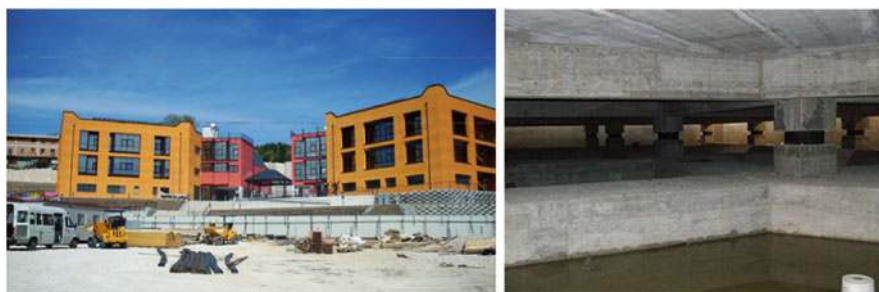
Fig. 14.15 Left : the isolated complex including the new Francesco Jovine primary school and “Le Tre Torri” Poly-Functional Centre in San Giuliano di Puglia (Campobasso), in 2008. Right : view of some the isolators supporting their common base slab
