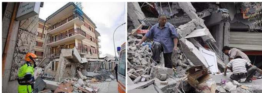
Fig. 14.26 Left : the “Student House” in L’Aquila, collapsed during the Abruzzo earthquake of April 6, 2009 ( M=6.2 ), causing the death of eight students. Right : secondary school in Dujiangyan (P.R. China), collapsed during the Wenchuan earthquake of May 12, 2008 ( M\approx 8.0 ), causing the death of 900 students
