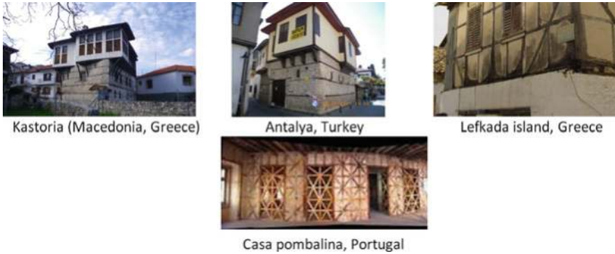
Fig. 8.8 Various types of timber reinforced structures in Europe (Source: https://www.google.gr/search?q=casa+pombalina+lisboa )
