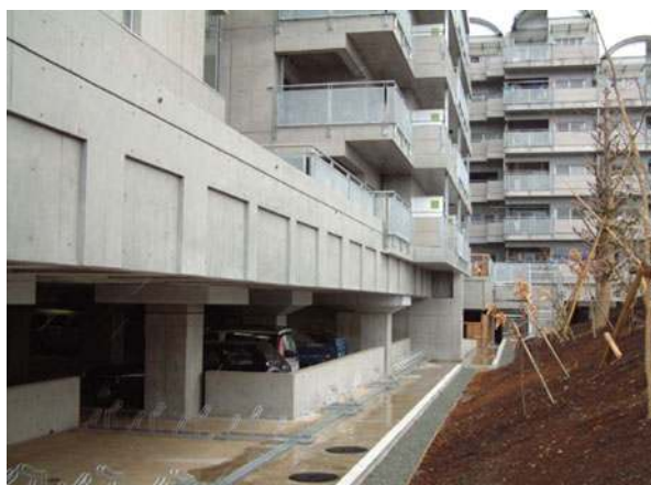
Fig. 14.6 Lateral view of a complex of twenty one 6- to 14-storey buildings, all erected on an unique “artificial ground” isolated at Sagamihara (Tokyo area) with 48 LRBs, 103 SDs and 83 BBs (Martelli and Forni 2010). This was the first Japanese application of “artificial grounds”
