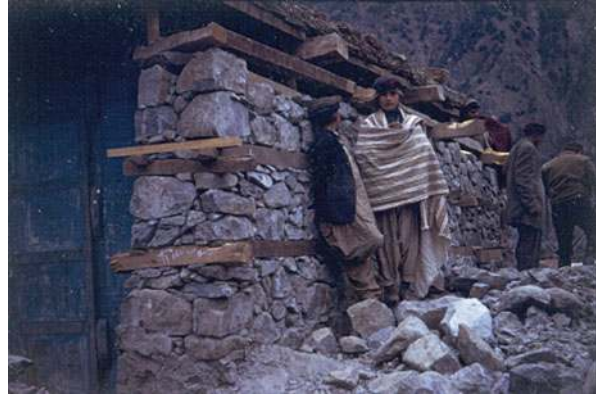
Fig. 1.8 Stone masonry buildings with roofs supported on timber columns independently of the walls, from UNESCO mission to 1974 Pattan earthquake (Ambraseys et al. 1975)
