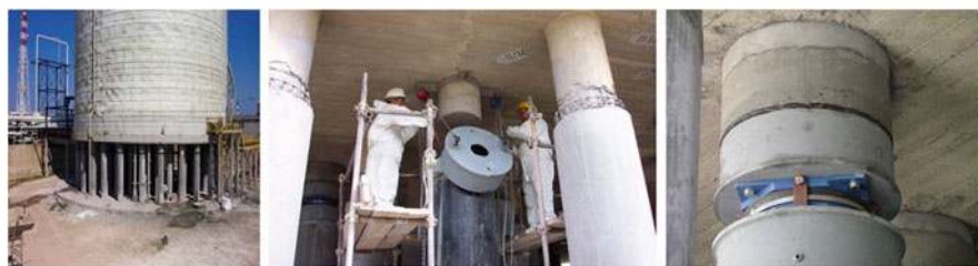
Fig. 14.16 One of the three tanks of the Company Polimeri Europa of the Italian ENI Group located in Priolo, which were seismically retrofitted using U.S. FPS devices in the years 2005–2008 and one of the isolators during and after its installation. To the knowledge of the authors, this is the only application of SI to chemical plants and components so far existing in Italy (prior to the 2009 Abruzzo earthquake, it was also the only application of CSS devices in Italy)
