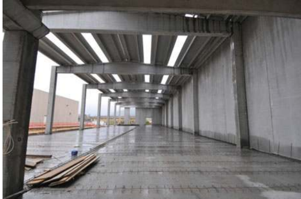
Fig. 4.1 Undamaged structural system of the precast industrial building after the L'Aquila 2009 earthquake
