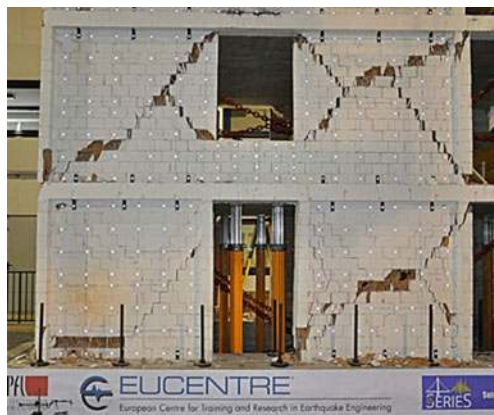
Fig. 12.16 URM walls of shake table test unit after Run 9 (Beyer et al. 2014)
