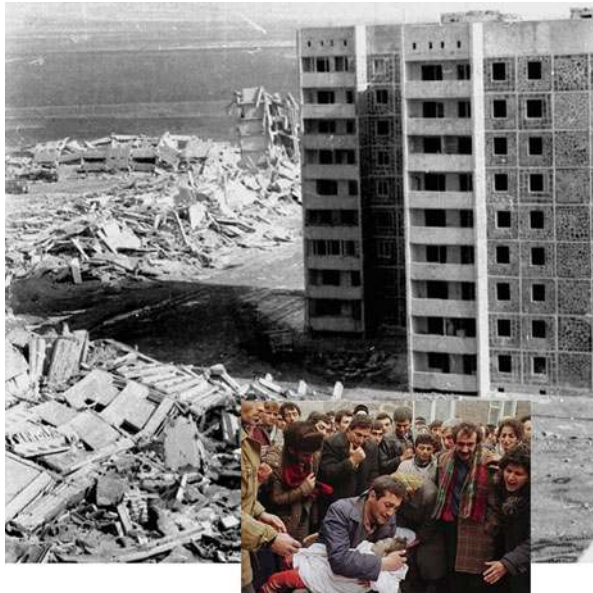
Fig. 4.2 Large panel precast structure standing among the rubble of the precast frames, which caused a terrible tragedy during the Spitak 1988 earthquake
