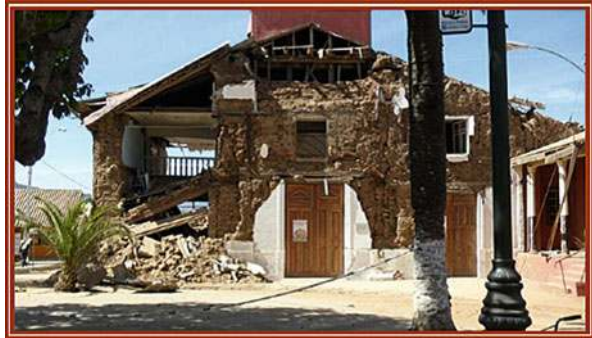
Fig. 1.15 Investigation of the performance of strengthened historical structures formed part of the EEFIT reconnaissance following the 2010 Maule Chile earthquake (Lubkowski 2010)
