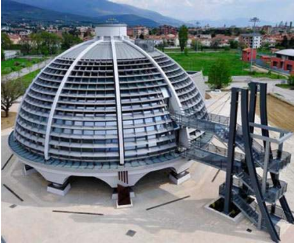
Fig. 14.17 Main building of the Civil Defence Centre of Foligno (Perugia), former seismic zone 1, isolated by 10 HDRBs and certified as safe by A. Martelli in 2011
