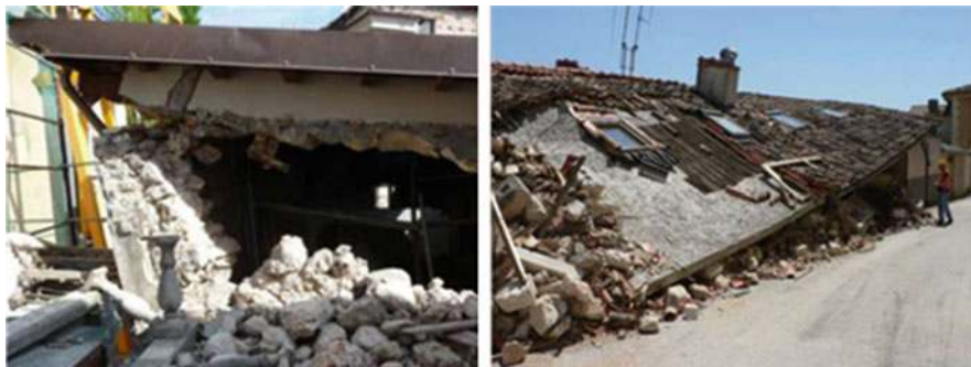
Fig. 8.30 Catastrophic effect of RC slabs on poor quality (unstrengthened) masonry (courtesy of Prof. C.Modena)
