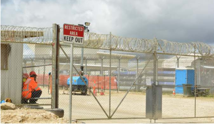
FIGURE 9. PNG LNG project site. Photo by Kenneth I. MacDonald.
