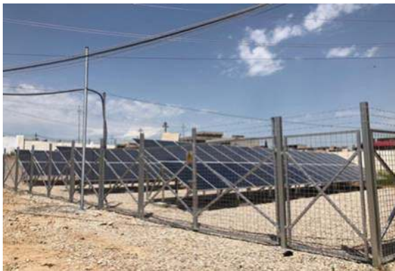
Figure 8.2 Solar-powered water project in Shekhan.
