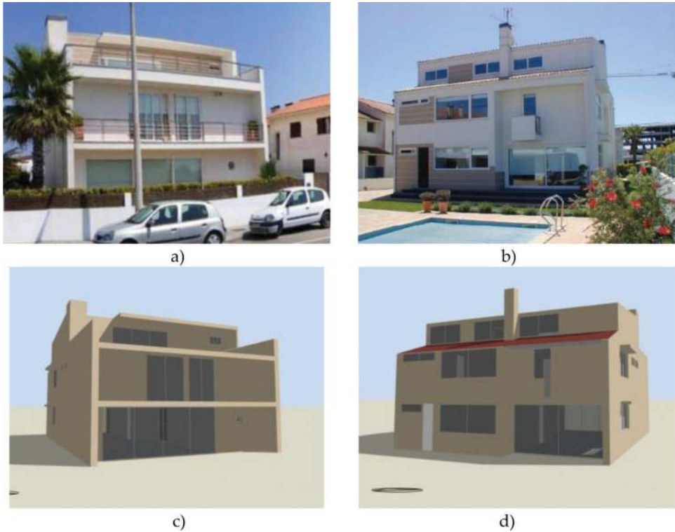
Figure 18. LSF residential building and DesignBuilder model [9]. (a) Front view. (b) Rear view. (c) Front view. (d) Rear view.
