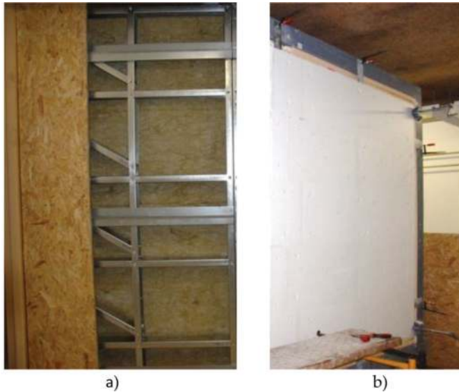
Figure 12. LSF wall tested in a climatic chamber [27]. (a) Inside view of the LSF wall structure. (b) External thermal insulation (EPS).
