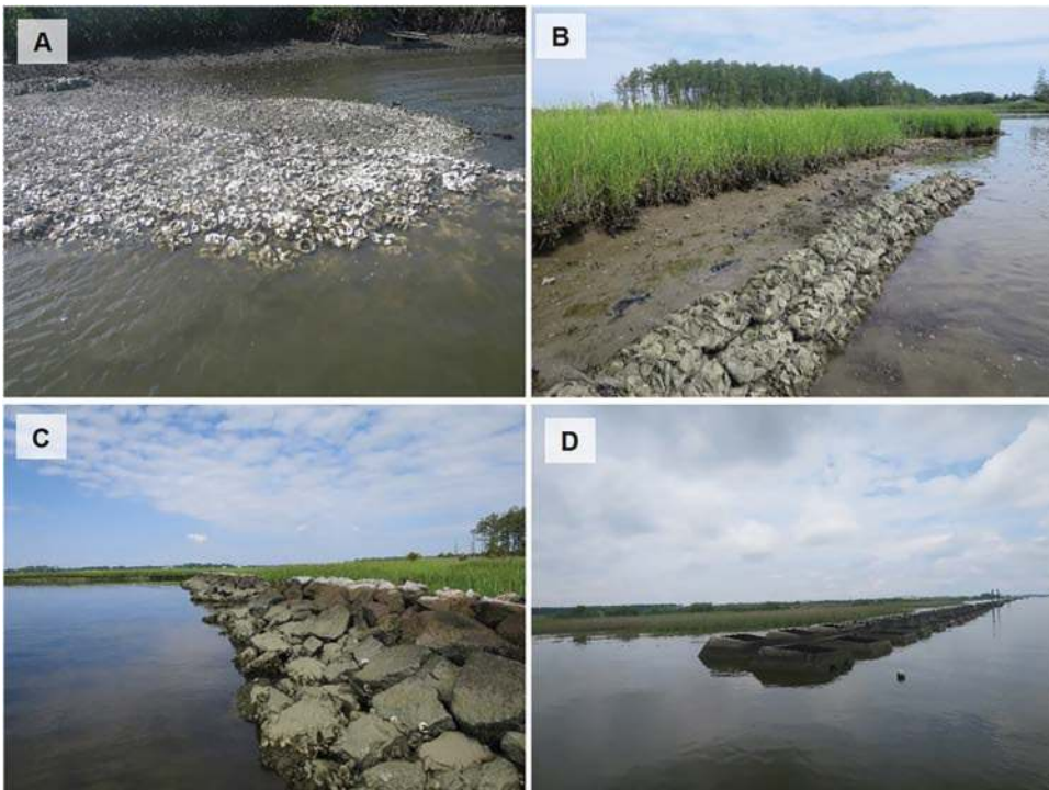
Figure 8 Examples of living shorelines projects along the East and Gulf coasts, United States. (A) Restored oyster reefs using oyster mats; (B) bagged shell oyster reef living shorelines with saltmarsh; (C) rock sill with saltmarsh and (D) wave-attenuating units with saltmarsh.
