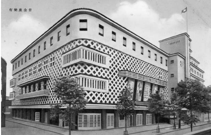
Figure 3.55 Exterior of the Yuraku-za theatre, opened in 1935.
