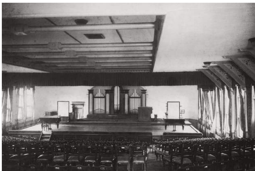
Figure 3.7 Interior of the auditorium of the Tokyo Academy of Music. The photo shows the auditorium in 1930, with the enlarged stage and free standing wooden chairs with only the seats upholstered with leather.
