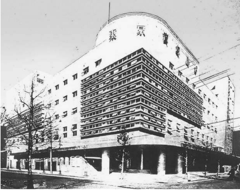
Figure 3.52 Façade of the Tokyo Takarazuka Theatre, located across the street to the north of the Imperial Hotel.
