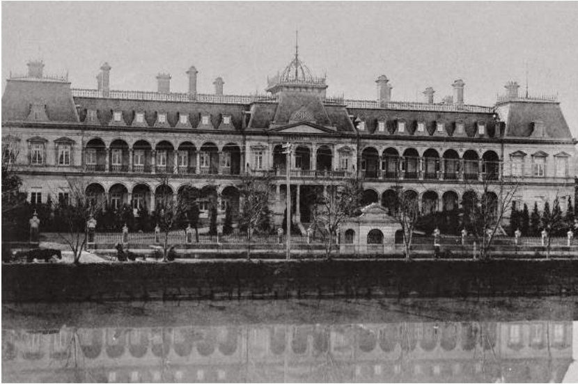
Figure 3.11 Façade of the Imperial Hotel, which opened in 1890. The moat seen in front of the hotel later disappeared and a street took its place. The architectural style was described as a “three storey timber construction in a German meets French Second Empire Beaux Arts style” (Lloyd Jones 2017).
