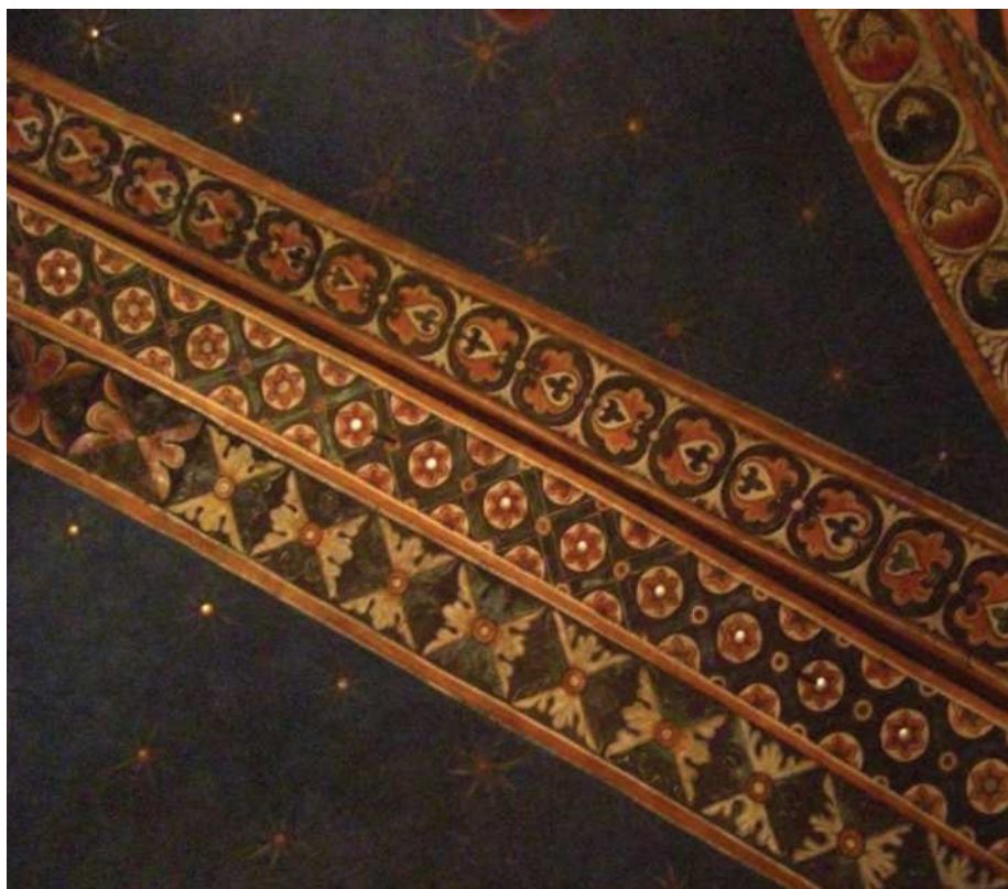
Figure 2.5: Ceiling of Lower Church with light reflecting off silver-backed glass insets, Lower Church, San Francesco, Assisi. Source: Author.
