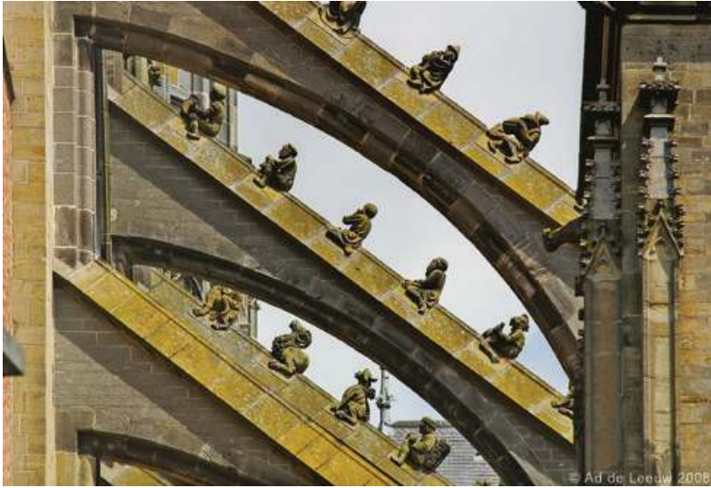
Fig. 12.4 Detail of flying buttresses of St John, 's-Hertogenbosch. Photos taken in June, 2016. Photo © Steve Whitmarsh
