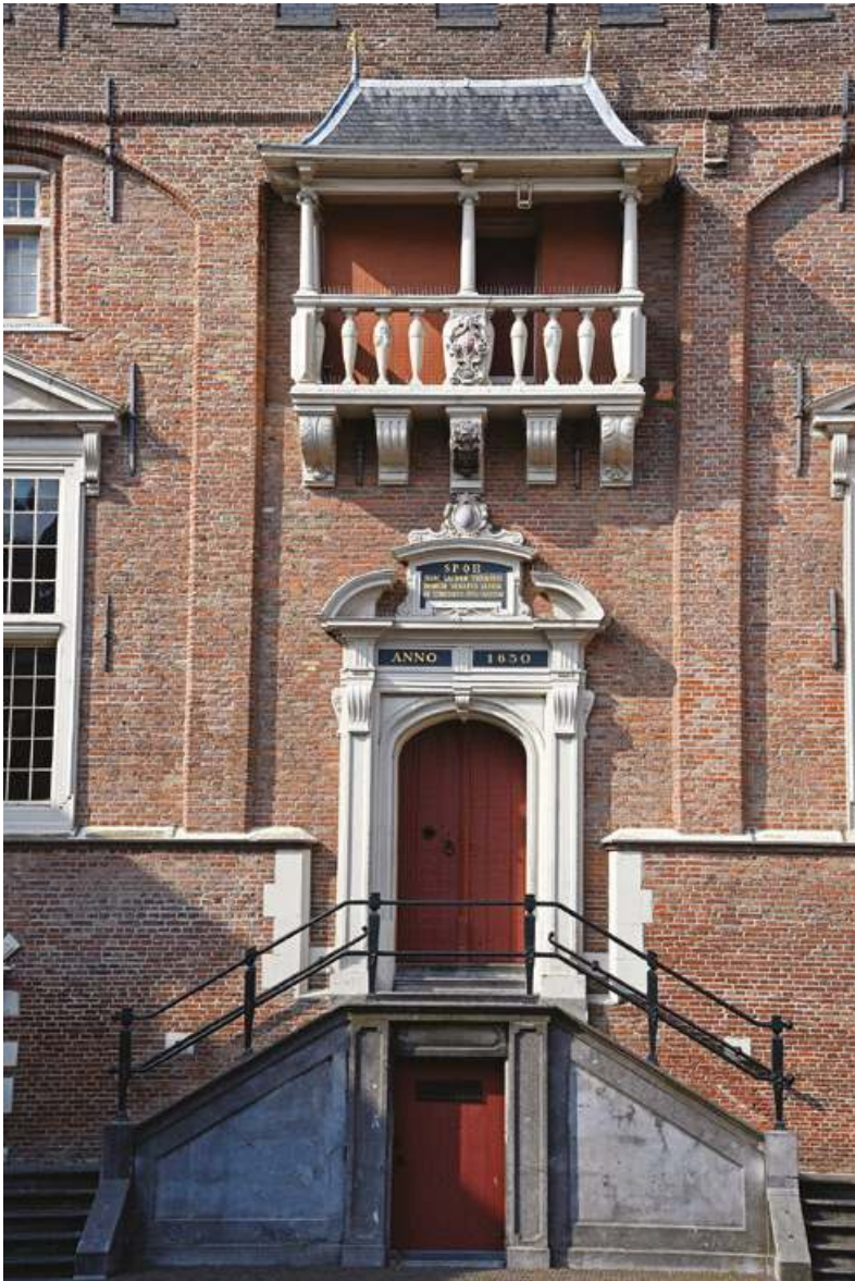
Fig. 12.8 Town hall, Haarlem, The Netherlands. Photo © Arco Images GmbH/Alamy Stock Photo
