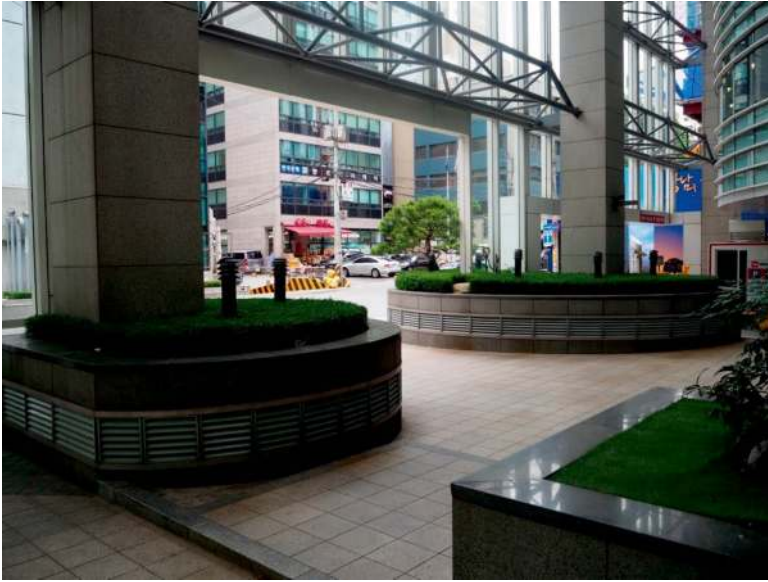
Figure 7.8a Photographs for POPS Case 2: POPS with piloti structure
