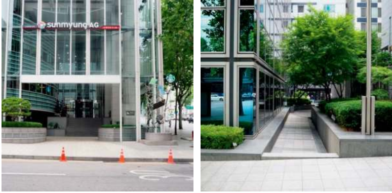
Figure 7.8b, c Photographs for POPS Case 2: Entrance to POPS with piloti structure and second corner POPS
