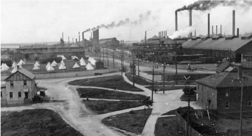
Sydney Steelworks, Nova Scotia. Steelworks during the 1923 strike (Courtesy Beaton Institute).
