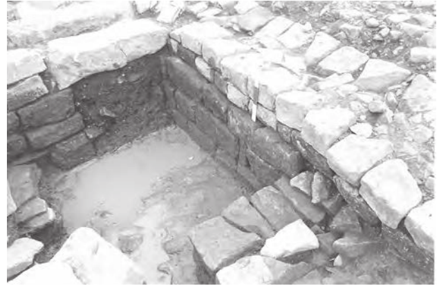
Fig re 7 The latrine cess pit from the north east side wing the outlet opening the large masonry of the pit side walls and offset for the hospital walls.
