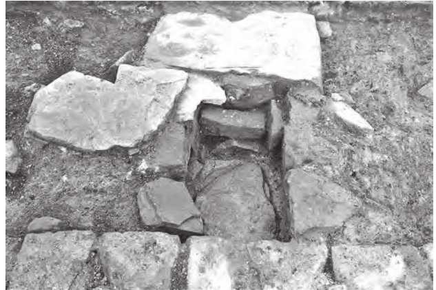
Figure 9.10: 'Drain/soakaway' N12:58 from the west.
