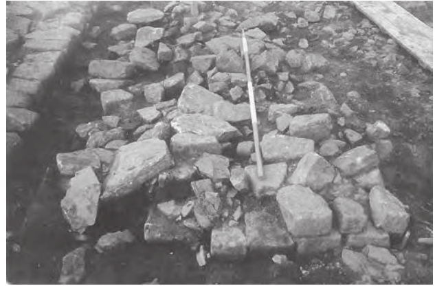
Figure 9 Hospital demolition rubble E11:09 (from south).
