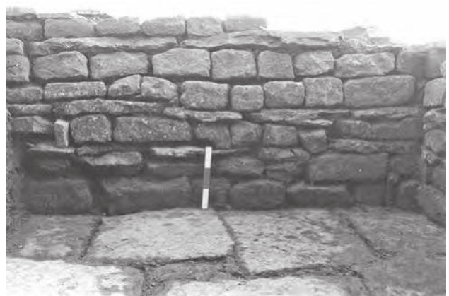
Figure 9.08: South wall of the courtyard cistern (N11:11).
