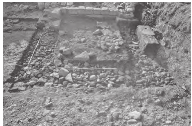
Figure 17.06: The primary floor base and foundations of the west gate's south guard chamber.
