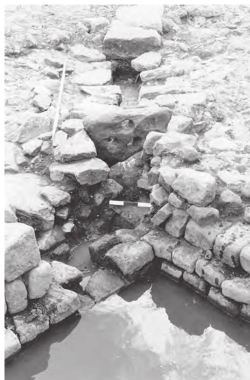
Figure 8 The water channel at the south west corner of the cistern with the filter stone apparent in the channel.
