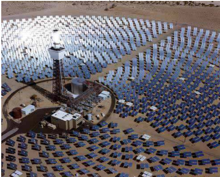
Fig. 21. (a) Schematic of a power tower. Image adapted from Energy Efficiency Renewable Energy Network {J. Tidwell, 2005} [61]; (b): Solar Two, power tower. Image courtesy of NREL's Photographic Information Exchange [62].
