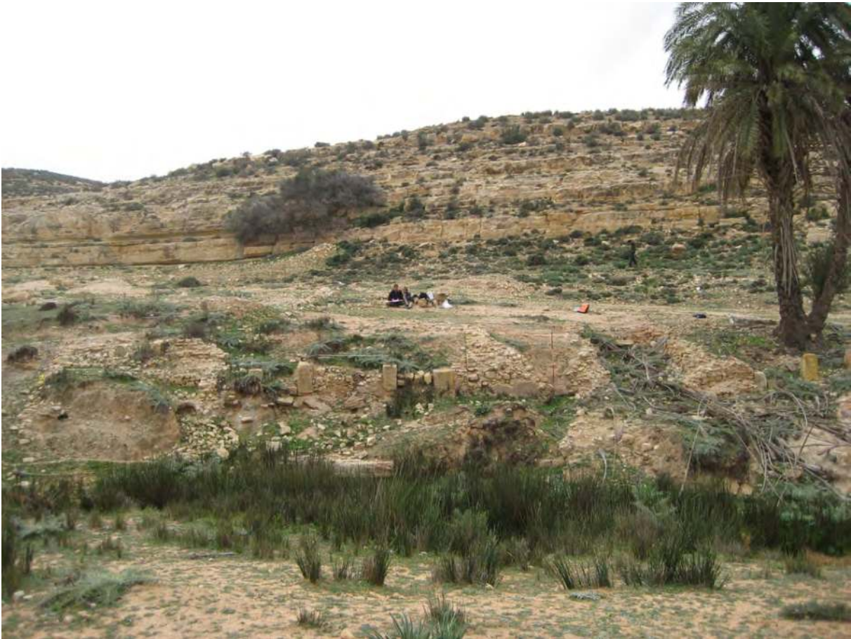
Figure 3.36: A general view of Ain Guman villa and bath (GUM87) showing the eastern wall constructed in opus africanum.
