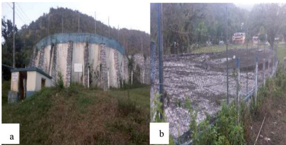
Figure 2. (a) An elevated rainwater concrete catchment of Elisabeth, Jamaica; (b) the surface runoff and the storage tank of Elisabeth, Jamaica RHI. (Adapted from Betasolo and Smith, 2017.)
