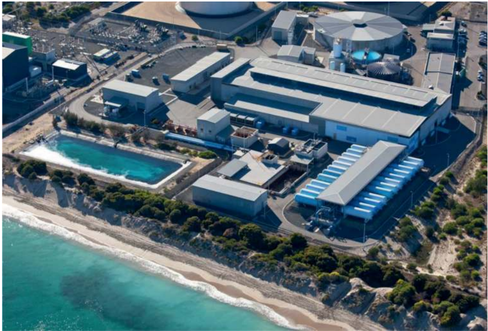
Figure 5. Perth desalination plant.
