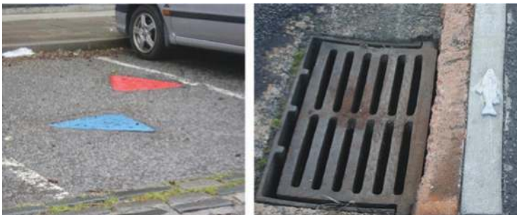
Figure 17.16 Trying to prevent pollution from misconnections or casual disposal into the wrong drain.
