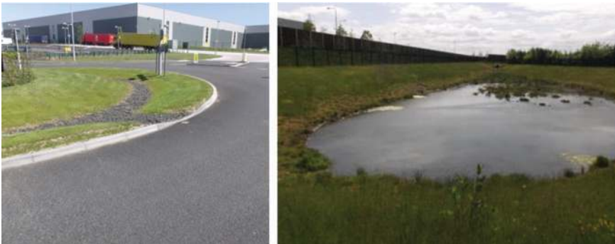
Detention basin prior to retention pond fed by linear wetland/swale and filter drain network, DEX Dunfermline, Scotland
