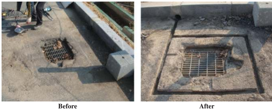
Figure 12.14 A flow diversion channel was constructed to ensure flow diversion to the hybrid constructed wetland as part of the non-routine maintenance.
