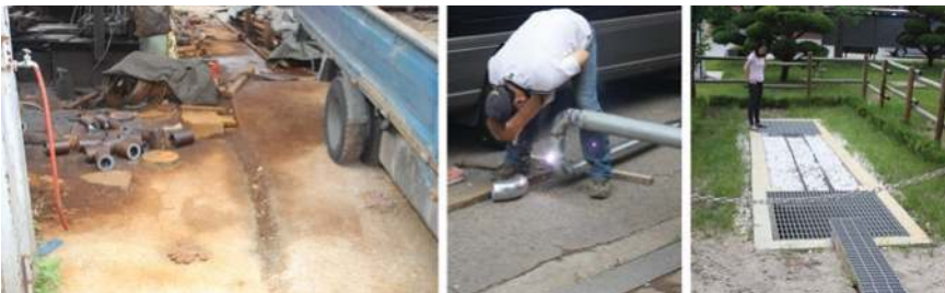
Figure 17.11 Sources of day to day contamination by toxic metals, and BMP system for capture.
