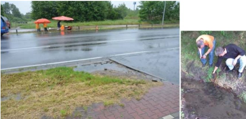
Above: under-drained grass swale under investigation for long term effectiveness at Hoppegarten (photo credit Harald Sommer). Below: Original outlet from Hoppegarten development: still the only discharge point to small receiving watercourse.
