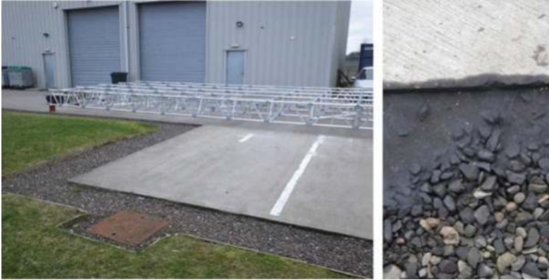
Figure 17.17 Surface drainage using gravel trenches allows for easy detection of poor practice disposal and leaks. Also provides a first stage of degradation for lesser levels of contamination by microbes on the gravel.
