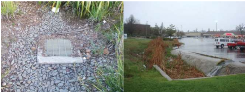
Figure 12.2 Bad management: overflow pipe in bioretention ( above left ) and small constructed wetland ( above right ) blocked with litters (San Francisco/California).
