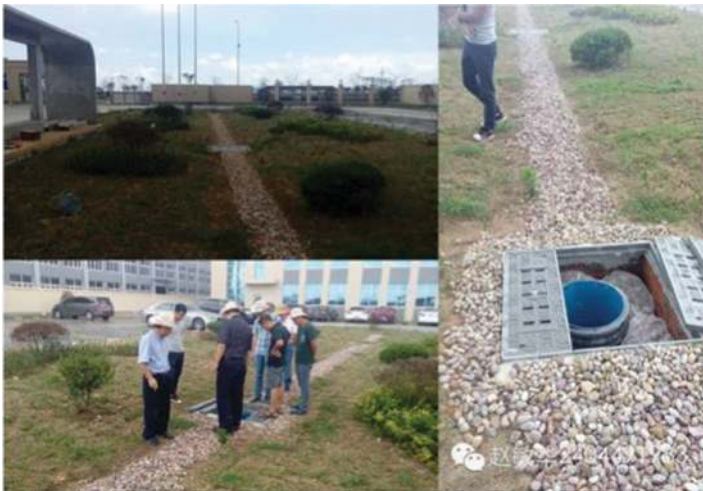
Figure 8.7 Rain garden and infiltration trench in the campus.
