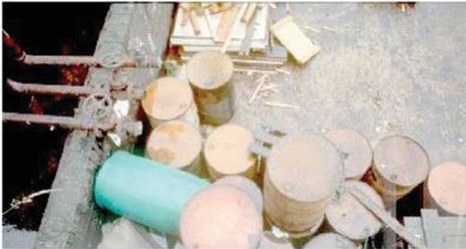
Figure 17.4 Empty drums and various wastes presenting pollution risks.
