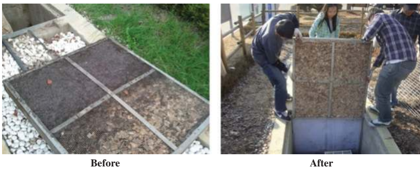
Figure 12.9 Woodchip in the vertical media cartridge was replaced as part of the non-routine maintenance in the infiltration trench.
