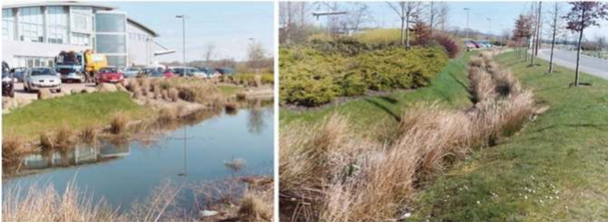
Source and Site controls (filter strip and pool), feeding head of a conveyance swale, J4M8
