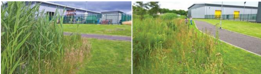
Figure 9.4 Conveyance swales, Clyde Gateway Industrial Estate, Scotland, UK.
