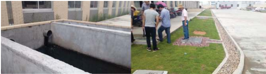
Figure 8.8 Rainwater harvesting system: pre-treatment and storage tank.
