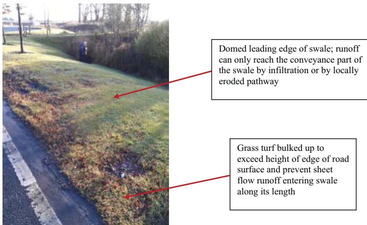
Figure 11.4 Some British builders were not familiar with swales; an unfortunately 'domed' section of grass swale at part of J4M8 business park.
