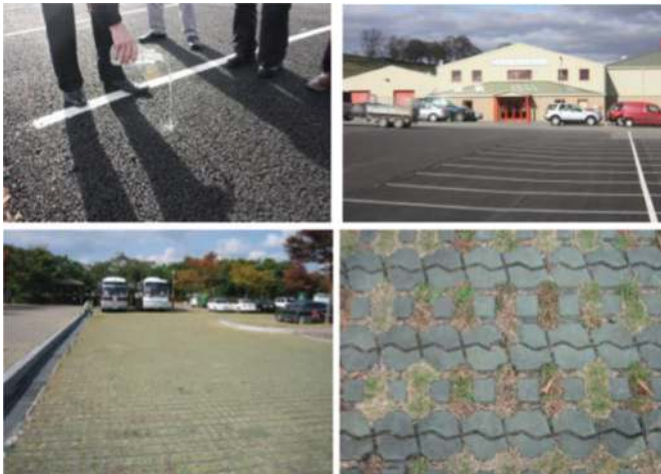
Figure 9.8 Above: Permeable blacktop serving the car park for a meat trading market near Dingwall Scotland, UK. Below: Hybrid concrete/grass permeable surface, with exceedance flow collection drain, serving a coach and car parking area at a water utility installation in South Korea.
