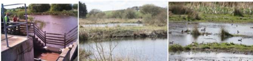
Figure 9.11 Retention pond in modular arrangement (3 ponds and a wetland) receiving runoff from a timber industries business park in Scotland, UK. Note the provision for management of incidents as well as day to day runoff. Swales or filter drains provide the source controls around the site.
