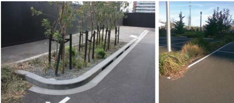
Figure 9.5 Above left: Bioretention feature, Melbourne Docklands, Australia. Right: Bioretention features taking car park runoff, Portland, USA.
