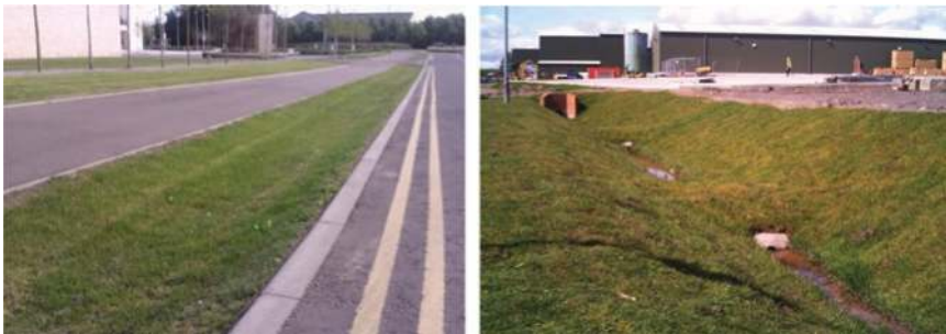
Figure 9.3 UK examples: Left (Photo credit Neil Mclean) Swale with sheet flow inlet over level kerb from road surface (Forth Valley, Stirling). Right : Grass swale with check-dams at Stephen's Croft, Lockerbie (timber industries development, 1990s).
