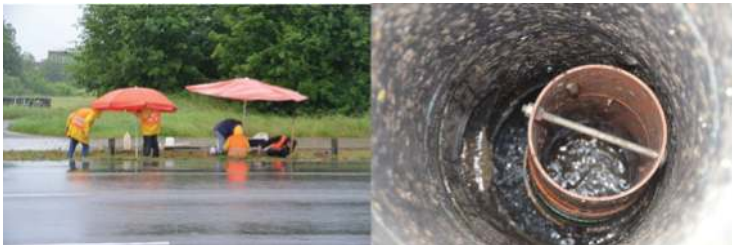
Figure 11.3 Soil sampling and permeability test in a swale, retention measure in manhole at Hoppegarten, Germany (Sommer, 2016).
