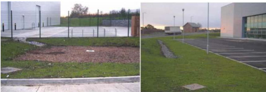
Figure 4.4 Examples of SUDS at industrial estates.
