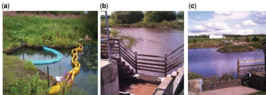
Figure 17.14 Oil spill containment at industrial estate discharge to a retrofit SUDS pond in Livingston, Scotland and (a) contingency design in inlet to treatment pond from swale network and (b) penstock valve at outlet from first pond (c) a timber industries development, Lockerbie, Scotland.
