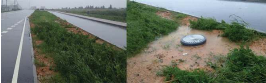
Figure 8.4 Bioswale in Jintang Road right after a 100-mm storm event.
