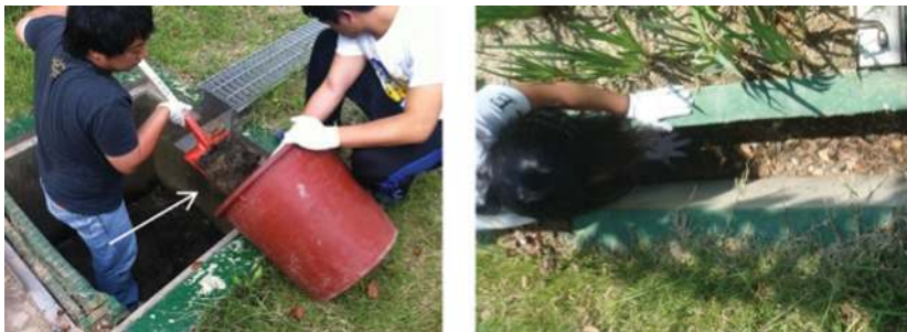
Figure 12.8 Sediments accumulated in the pre-treatment tank of the infiltration trench ( above left ) and overflow area of the hybrid constructed wetland ( above right ) were removed as part of the non-routine maintenance.
