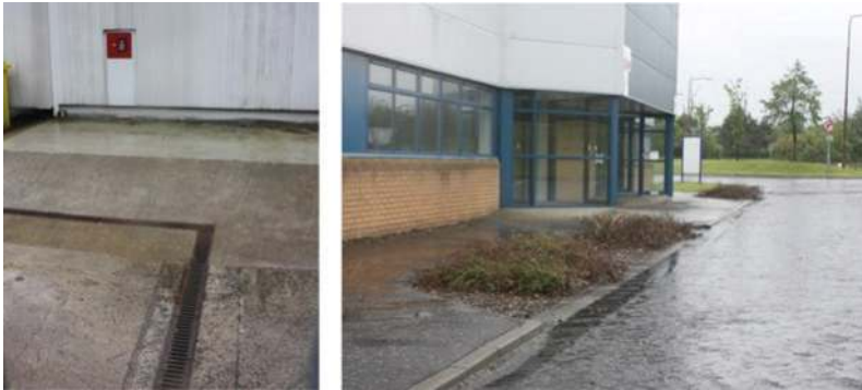
Figure 17.13 Demarcation and collection drain for higher risk outdoor yard area ( left ). Rain garden taking road runoff and providing visible treatment facility with reduced risk of direct contamination of water environment in event of a spill ( right ).
