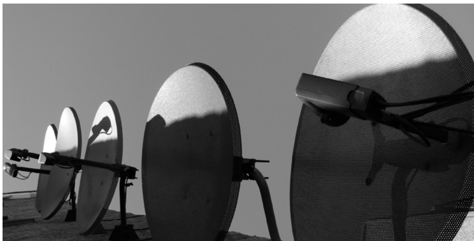
Figure 5.2 An array of satellite dishes. (credit: Matthew Colvin de Valle, Flickr)
