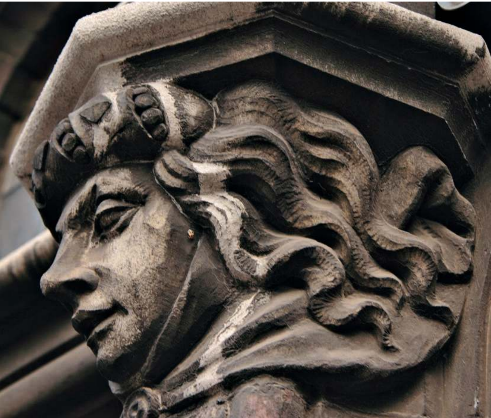
▲ Ornamental work embellishing the former Chemical and Pharmaceutical Laboratory on Hugo de Grootstraat
