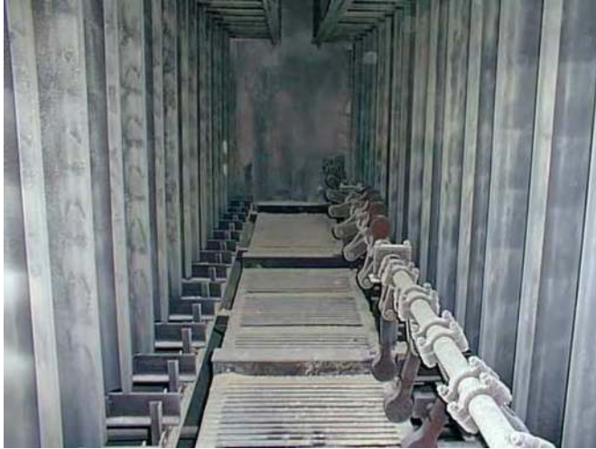
Fig. 2. Inner part of the ESP.
