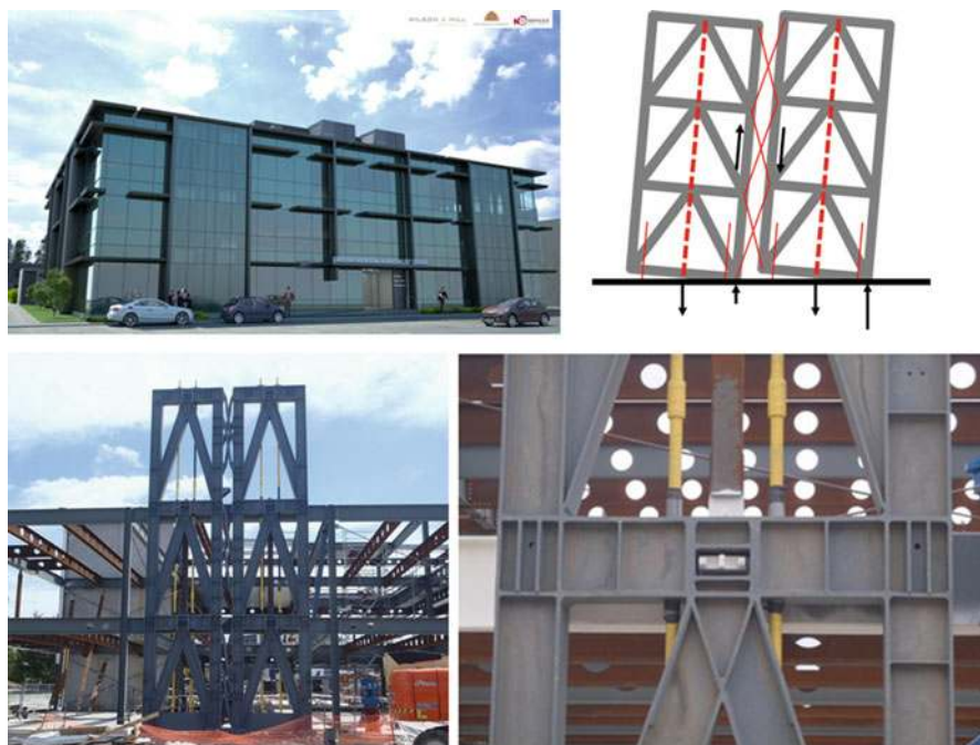
Fig. 13.34 Forté Health Medical Centre, three storey building with over 5,000 m 2 of specialist medical facilities. Post-tensioned steel rocking coupled ‘walls’ (or braced-frames) in both directions, combining hysteretic and viscous dampers in parallel for “an advanced flag-shape” system. Bottom right: secondary interior moment-resisting frames implementing a sliding hinge joint beam-column connection solution
