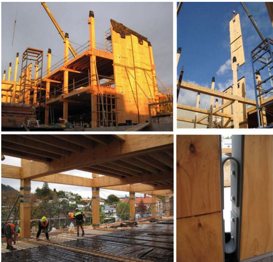
Fig. 13.27 Nelson Marlborough Institute of Technology, (NMIT), Nelson, New Zealand. Post-tensioned timber (Pres-Lam) walls coupled with UFPs (Structural Engineers Aurecon; Architects Irving-Smith-Jack, Devereux et al. 2011)
