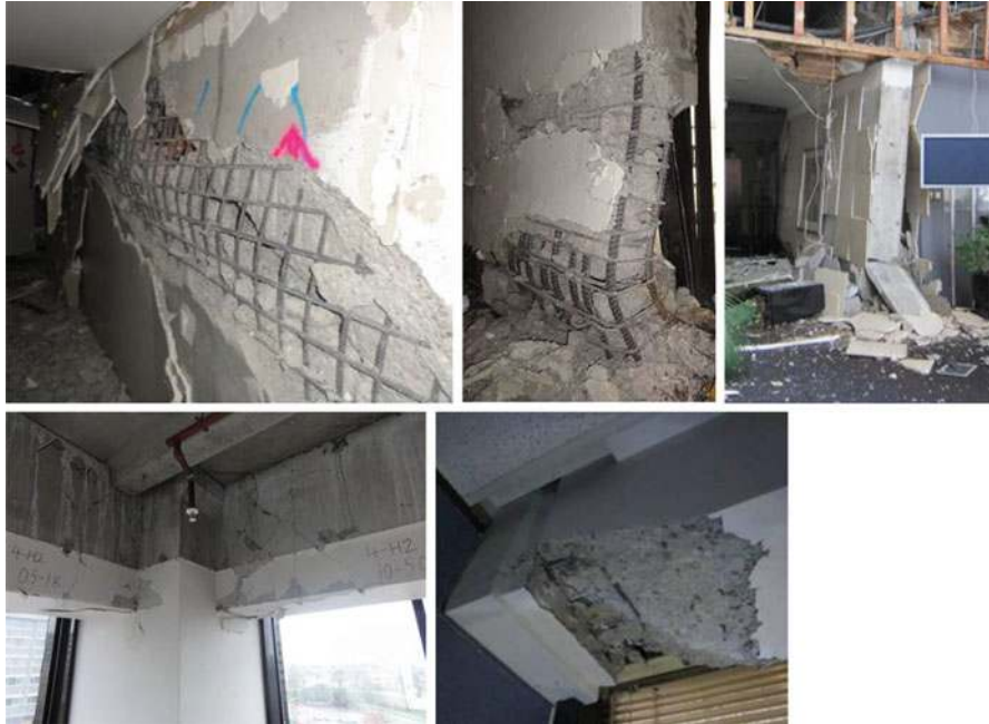
Fig. 13.3 Example of damage to RC frames and walls (all these buildings have been demolished) (From Kam et al. 2011; Pampanin 2012)
