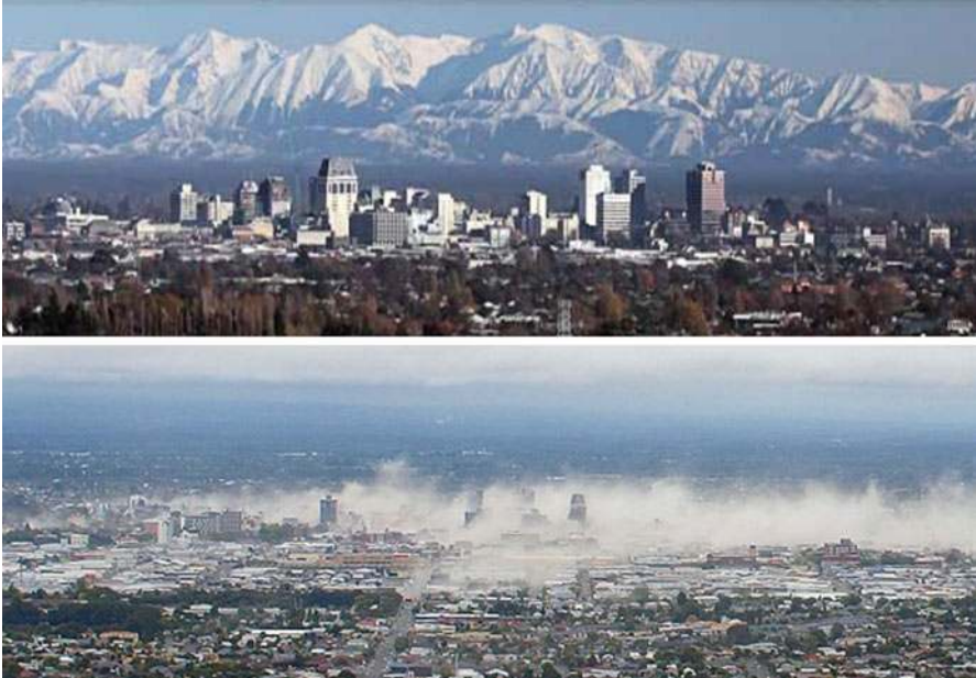
Fig. 13.1 Skyline of Christchurch CBD before ( Top ) and just after ( bottom ) the 22 Feb 2011 earthquake (Photo taken by Gilly Needham)
