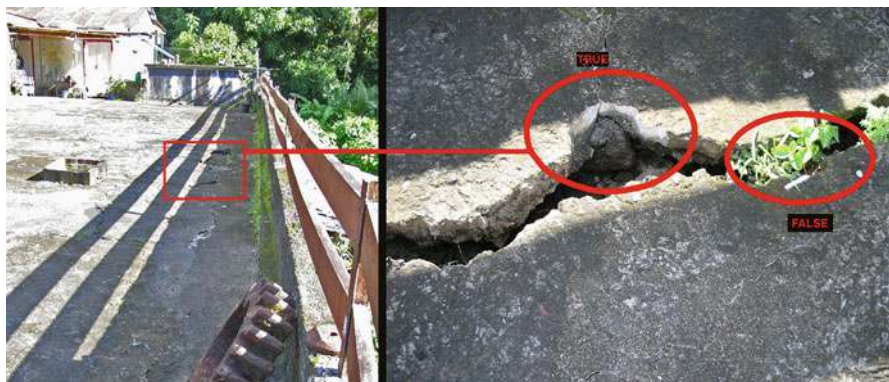
Fig. 16.6 False declaration by the inhabitants of terrace collapse (Les Saintes earthquake 2004). In fact the terrace is not collapse and it's only an increase of existing crack created by an amplification of differential collapse. We can see on the right picture the presence of vegetation in the crack, meaning the age of this damage
