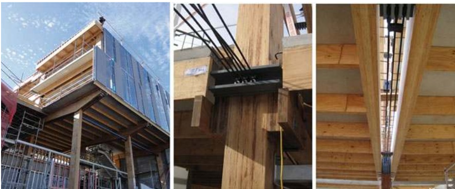
Fig. 13.30 College of Creating Arts – MacDiarmid Building, Massey University, Wellington, New Zealand. Post-tensioned timber (Pres-Lam) frames in the transverse directions with horizontal U-Shape flexural plate dissipaters on the first floor and Post-tensioned concrete (PRESS) walls in the longitudinal direction (Structural Engineers: Dunning Thornton Consultants)
