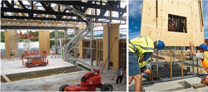
Fig. 13.28 Carterton Events Centre, New Zealand. Single-storey building with LVL truss roof (Designed by Opus International: Dekker et al. 2012)
