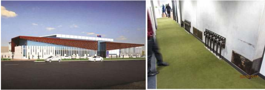
Fig. 13.26 Police Station in Rotorua. Post-tensioned concrete (PRESSS) walls with external & replaceable dissipaters in both directions (Structural Engineers: Spiire)
