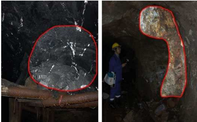
Fig. 9.8 Rockburst in underground mining
