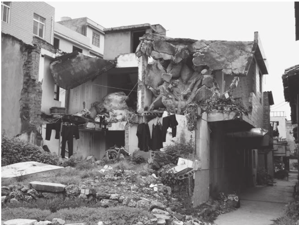
FIGURE 20. A partially demolished house. Photo by author.
