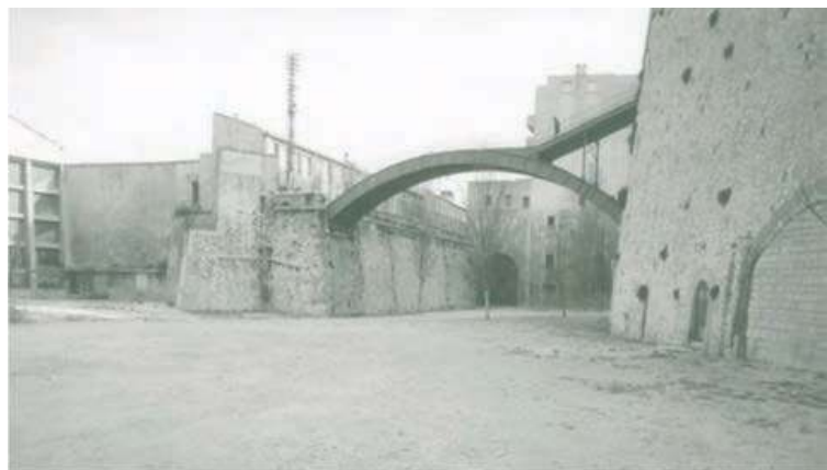
Probable ballast depot of 1824. (Photo by MTA, 1999.)
