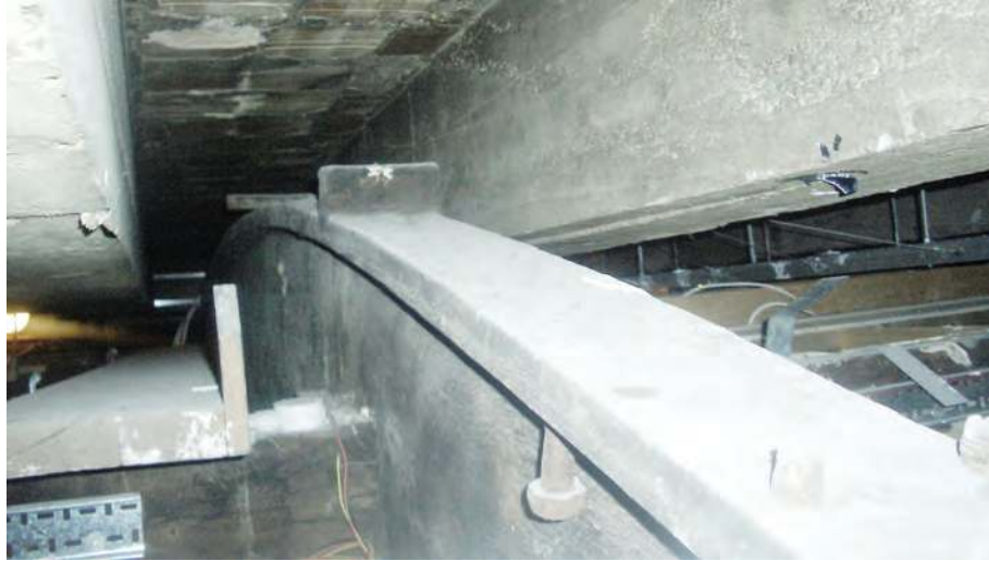
Fig. 20 The original 1848 Bramah and Robinson cast iron girders still exist today, bidden behind the plaster ceiling.
